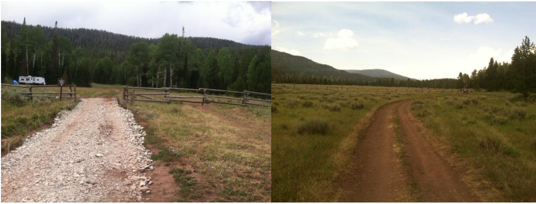
Road Repairs and fences used to control camping impacts and illegal ATV Use in the watershed
