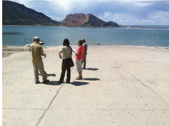
Boat Ramp Inspection at Antelope Flat, Flaming Gorge Reservoir
