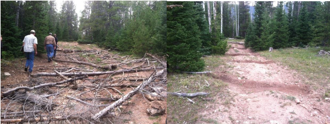
Road decommissioning and water-bars
