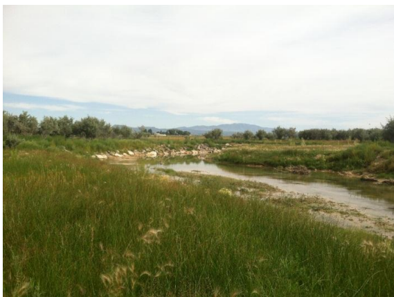
Sevier River Restoration work near Panguitch
