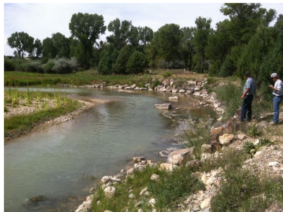
Sevier River Restoration work near Hatch
