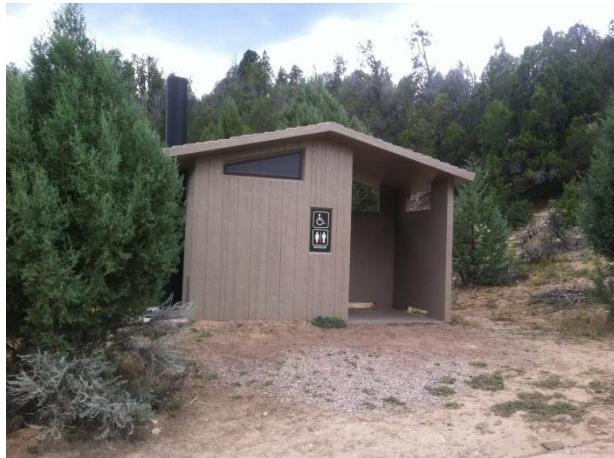
Outhouse constructed at trail head
