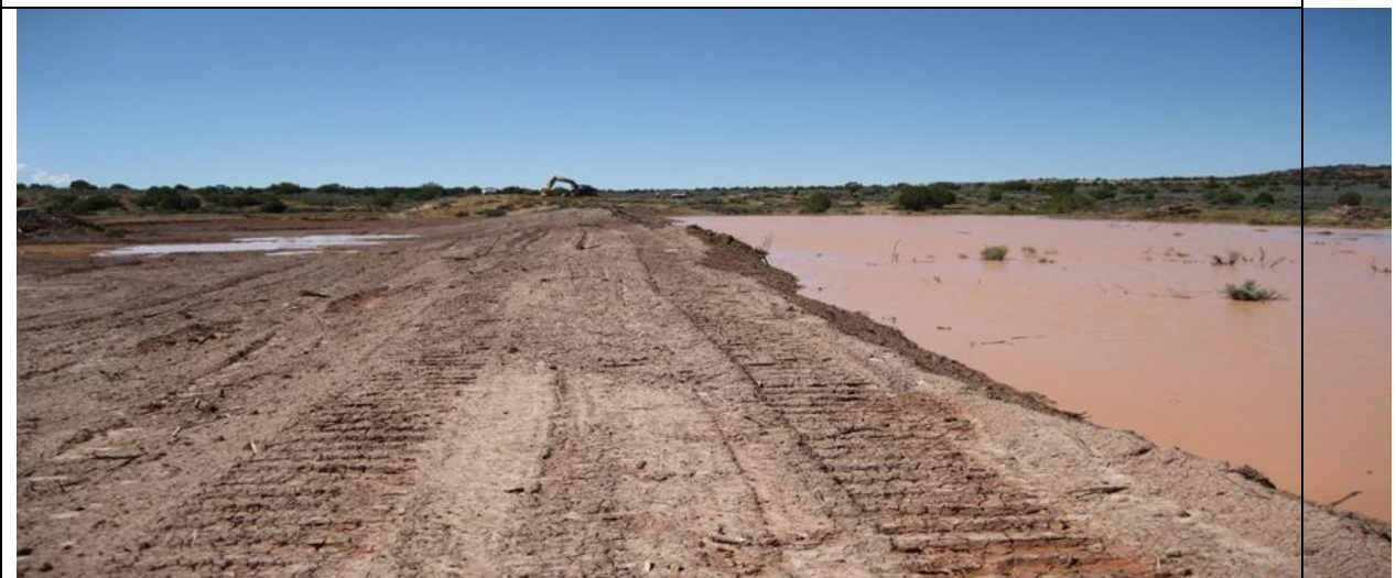
View of spreader dam & impounded runoff after monsoon rains.
